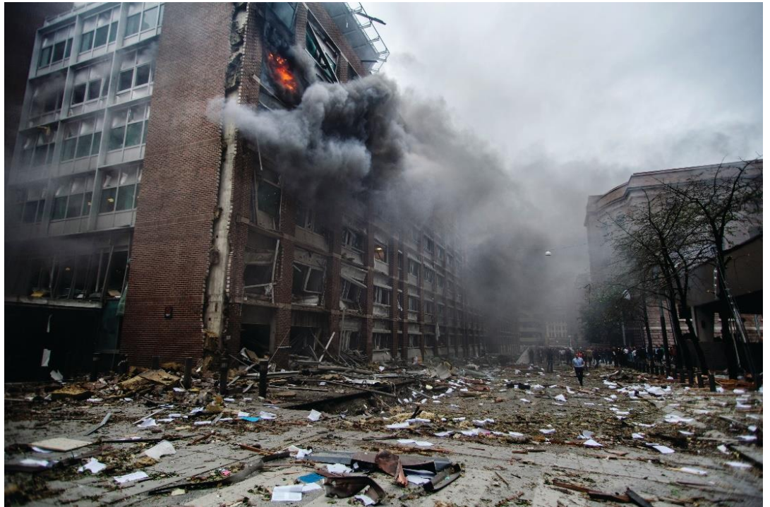
Grubbegata and Government Building 4, 22 July 2011. Photo: Fartein Rudjord
